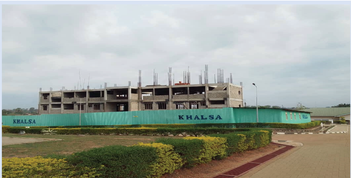
Figure 5: Administration Block Annex at Third Floor level (54% completion rate)
