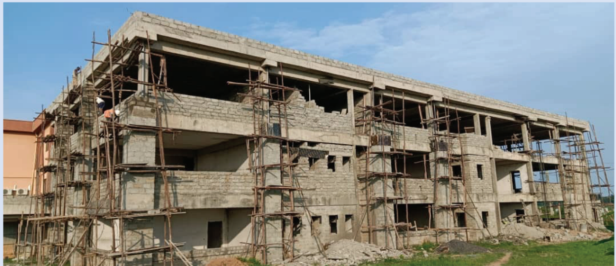
Figure 4: Health Science Laboratory Building at ring beam level (55% completion rate)
